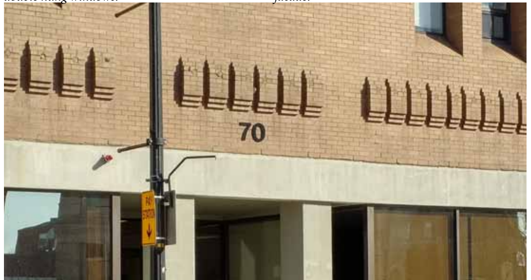
Taunton, MA: example of contemporary brick corbel detail in building facade and deep window sills
