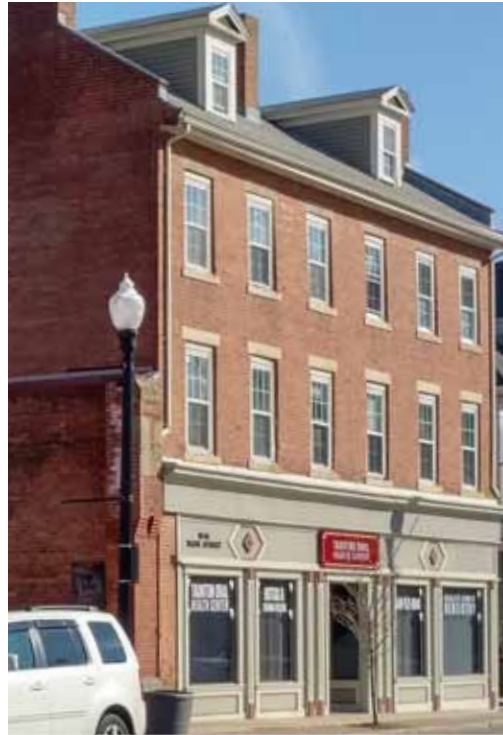
Taunton, MA: example of masonry lintels above double hung windows and masonry sills below double hung windows.
