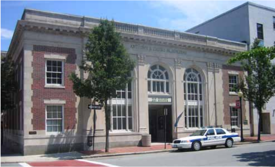
New Bedford, MA: example of stone quoins on the building corner, stone lintels above the double hung windows, stone sills below the window and keystones at the top of the arched windows.
