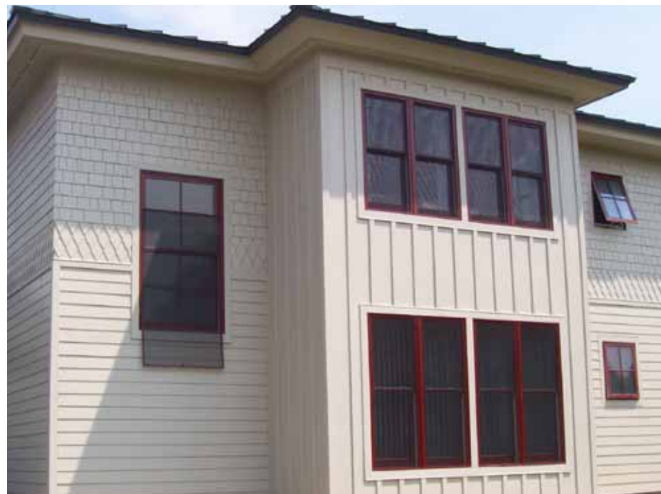
Example of standing seam metal roofing and fiber cement siding textures and patterns with complimentary color windows.
