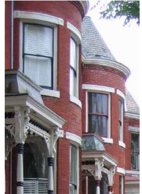
Richmond, VA: example of brick corbeling at roof eave and varying planes along the building facade.
