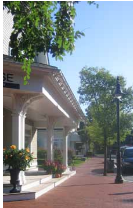
Plymouth, MA: example of architectural brackets supporting the porch roof overhang.
