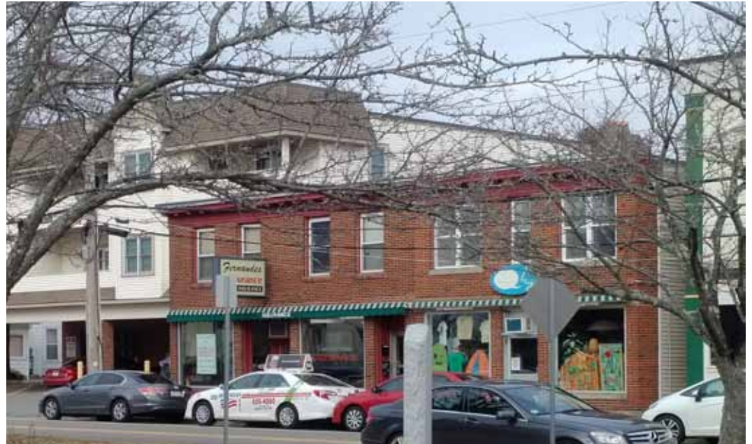
Stoughton, MA: example of double hung windows utilized on the second floor and storefront windows on the first floor. Avoid exposed mechanical systems in the storefront.
