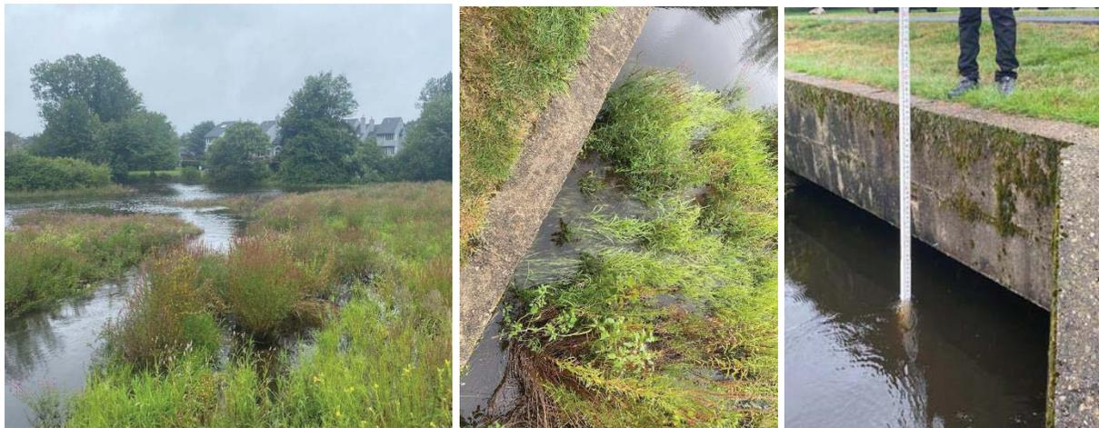
**Figure 2:** (Left) Main channel of Steep Hill Brook and vegetated floodplain; (Center) Evidence of high flows through floodplain and secondary box culverts; (Right) Culvert inspection of primary box culvert.
