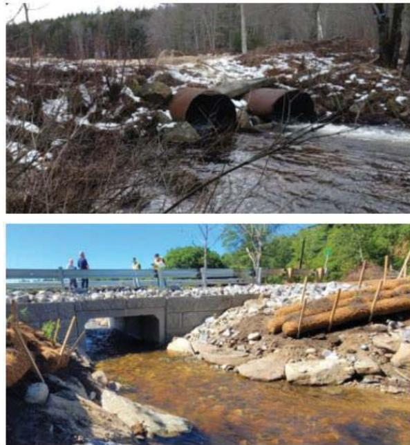
**Figure 6-4:** Culvert replacement example (Source: MVP)
