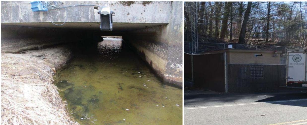
**Figure 2-3:** Example monitoring stations for flow (Left) and rainfall (Right) at Steep Hill Brook and Ames-Long Pond, respectively.
