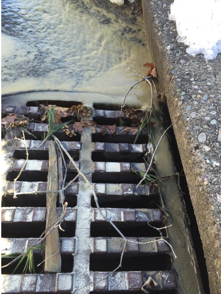
Inlet to Street Drainage system.
