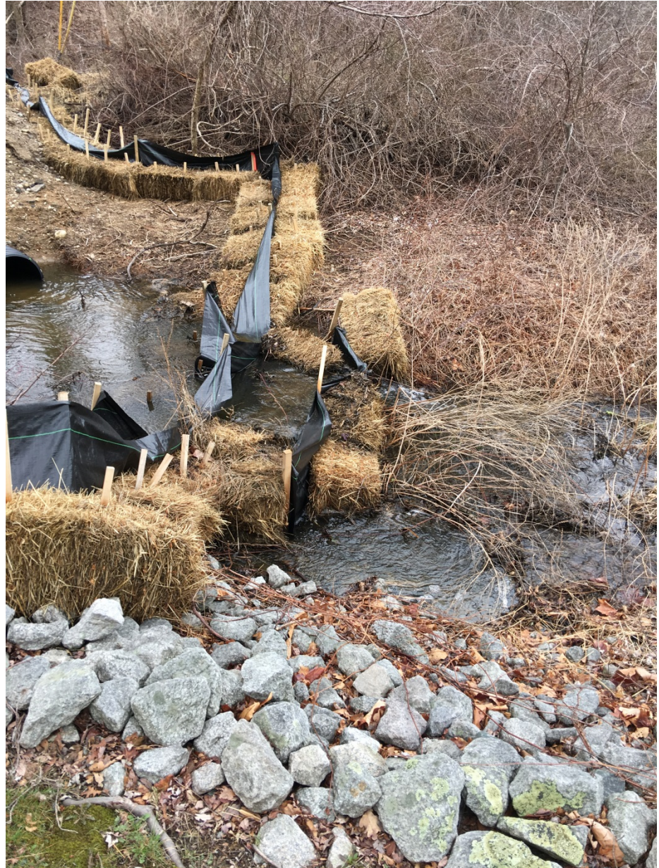
ECB or Erosion Control Barriers
