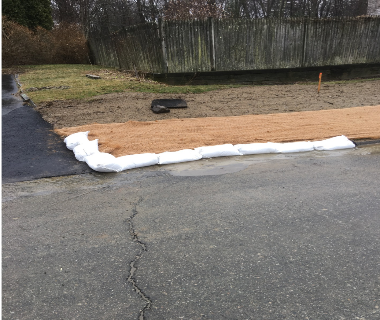
Jute Mat, BMP to prevent erosion until vegetated stabilization
