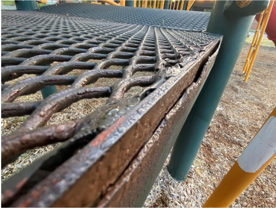
Deck delamination.
