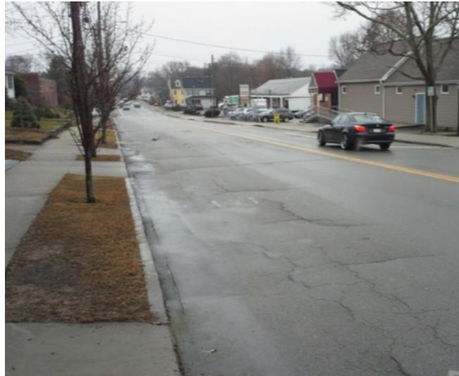
**Figure 3-11A: Moderate Cracking on Washington Street (Route 138)**
