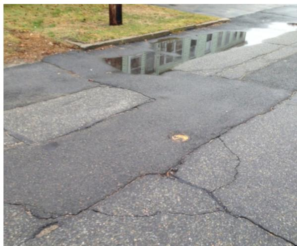
**Figure 3-11B: Dale Street - Significant cracking/patching, no sidewalk, ponding**
