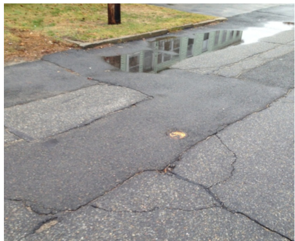
Dale Street - Significant cracking/patching, no sidewalk, ponding
