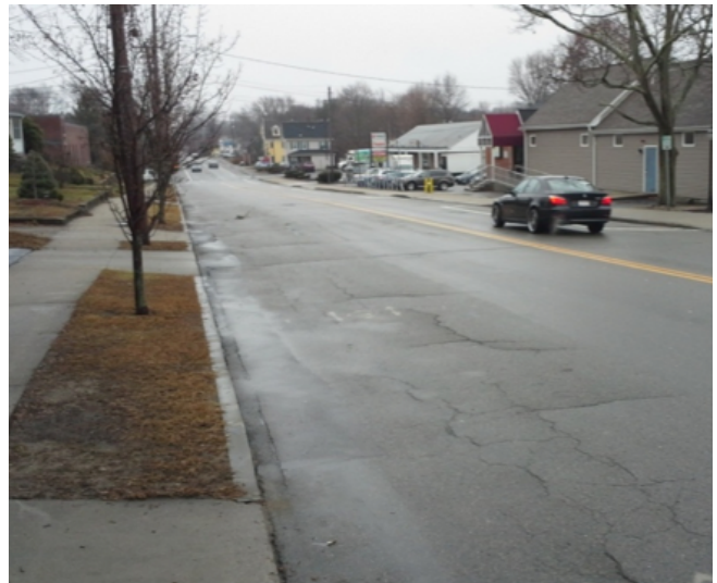
Moderate Cracking on Washington Street (Route 138)
